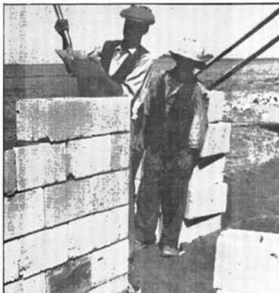
Here workmen are seen building a house at Dobsonville. The blocks are piled one upon another and sand is poured through the holes in the bricks. Mortar is used only at the window and door of the house.
