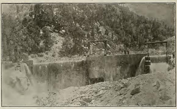
Diversion dam built by Llano del Rio colonists on Mescal Creek. Water is diverted from each side of the dam and this will flow into natural reservoirs to north and south of the dam.
